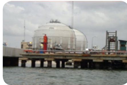
LPG SEA TERMINAL NAVGAS LTD. LAGOS, NIGERIA
